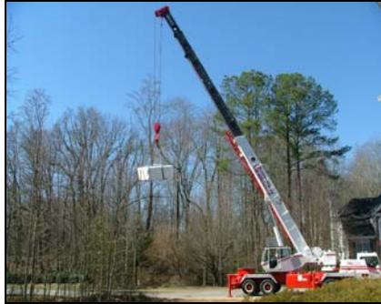
Other installations may require the use of special equipment to lift the spa from the delivery point to the installation location. Cranes and special equipment needs must be identified and pre-planned and scheduled long before the arrival of your spa.
